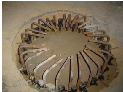
Figure 6. The SCC pile
