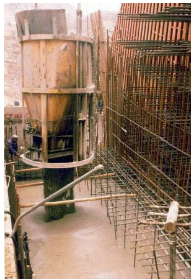
Figure 4. Orifice concreting
